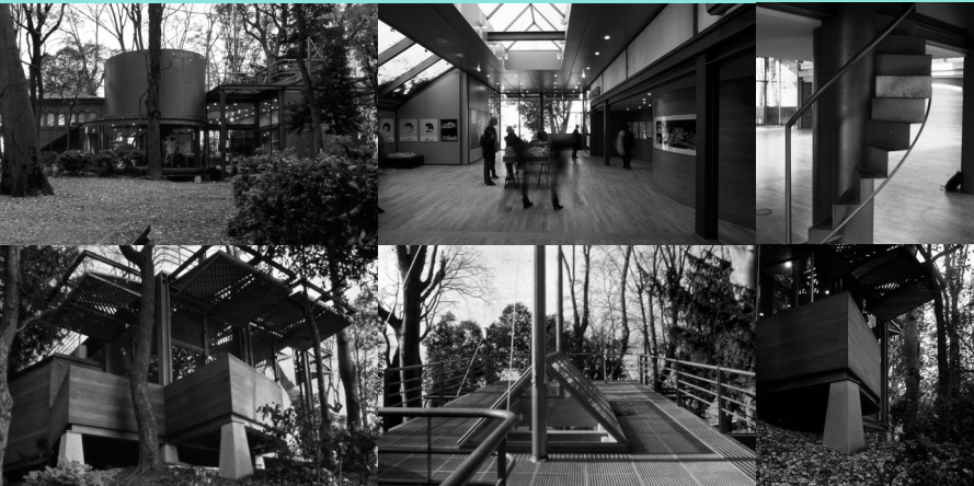
한국관 추가공사 Additional construction work on the Korean Pavilion, 1996.9.
